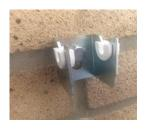
Wall Brackets - Offer up the radiator in the desired position, mark the bracket positions and fixing holes. The radiator should be placed a minimum of 10cm from the floor. Using the appropriate drill and fixings attach the brackets to the wall. After installing the plastic inserts into the hook part of the bracket the radiator can then be hung from the brackets.
